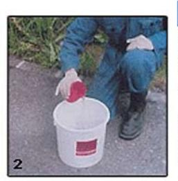
Now pour water in exact quantity into the mixing container using the measuring cup. Maintain the temperature of the mixing water under 20° C as far as possible.
