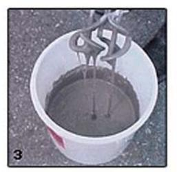
Mix the compound thoroughly with a mixer until a free flowing, lump-free mixture is formed.
