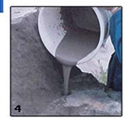
BETONAMIT R reached an expansion pressure of over 4,000 t/m2 in less than 10 hrs. The power of BETONAMIT R increases continuously thereafter and can, in this way. Reach an expansion pressure of over 10,000 t/m2 after approx. two days. However, an expansion pressure of 3,000 t/m2 is sufficient for most of the materials to be blown out!
